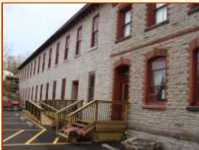
New paved parking and accessibility ramp at the MVTM, 2011
